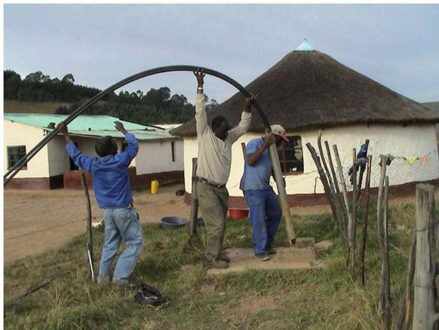
Figure 11: HPM Sipho Tenzo leading installation of a repaired Vergnet
