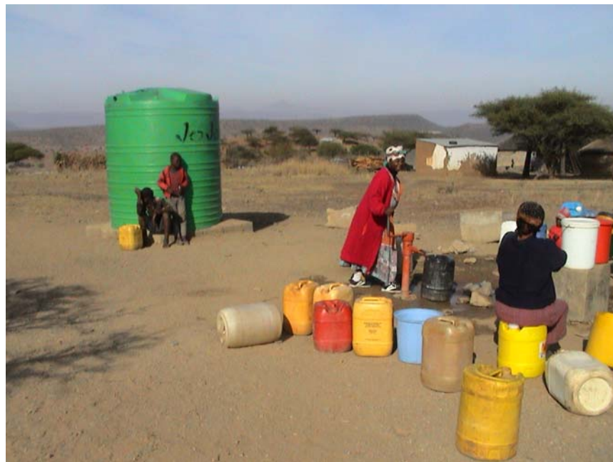
Figure 3: Handpump beside water tank for tankered water
