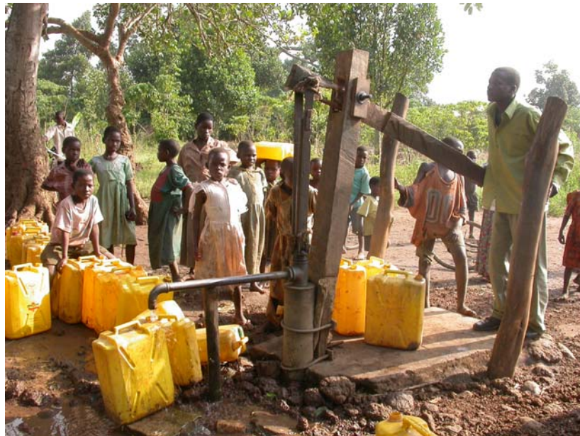
Figure 6: India Mark I handpump
