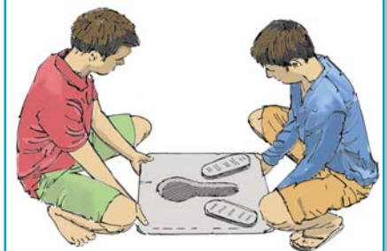
Figure 18. Lifting a sanplat
