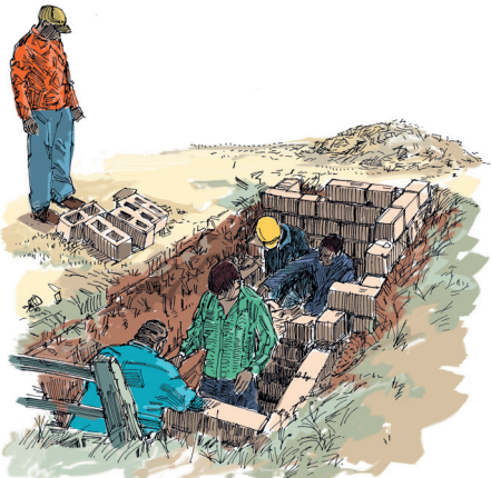
Figure 1. Lining from the base
