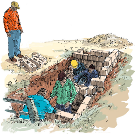
Figure 1. Lining from the base
