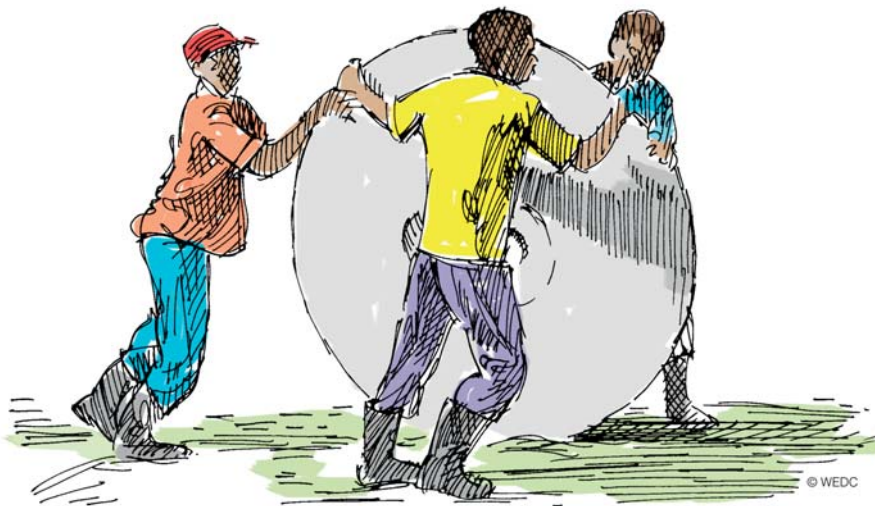
Figure 9. A circular concrete slab which can be rolled once cured is relatively easy to move from where it is constructed to its location over the pit.
