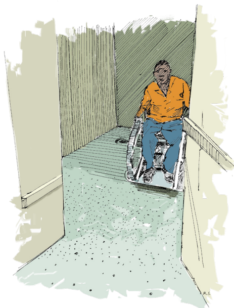
Figure 4. Latrine with a wide opening and enough space for a wheelchair to turn
