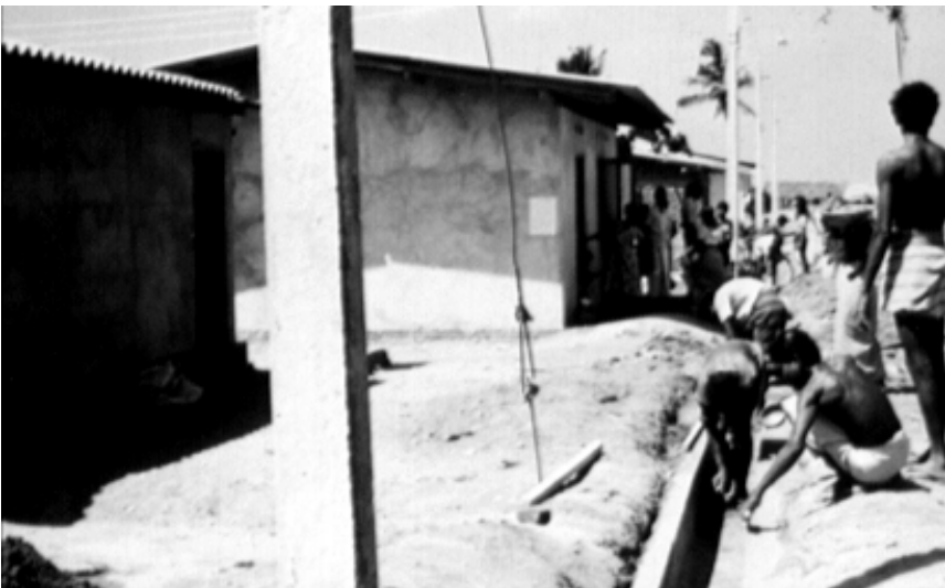
Photograph 3: Community management of neighbourhood drain construction in Colombo, Sri Lanka
