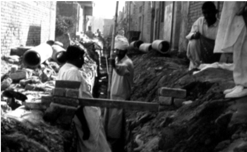
Photograph 6: Community management of sewer construction, Faisalabad, Pakistan
