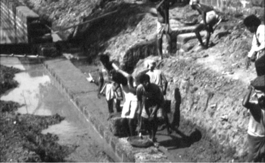
Photograph 2: Micro contractors improving secondary drainage, Cuttack, India
