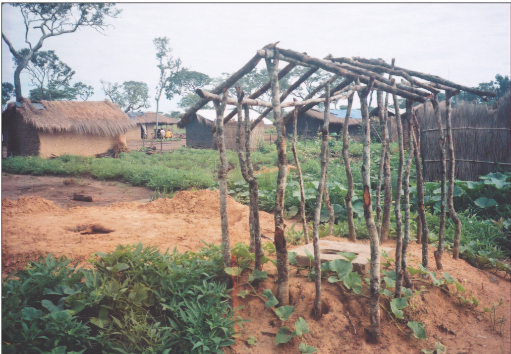
Family pit latrine under construction
