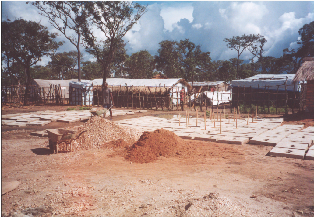
Preparation of concrete latrine slabs
