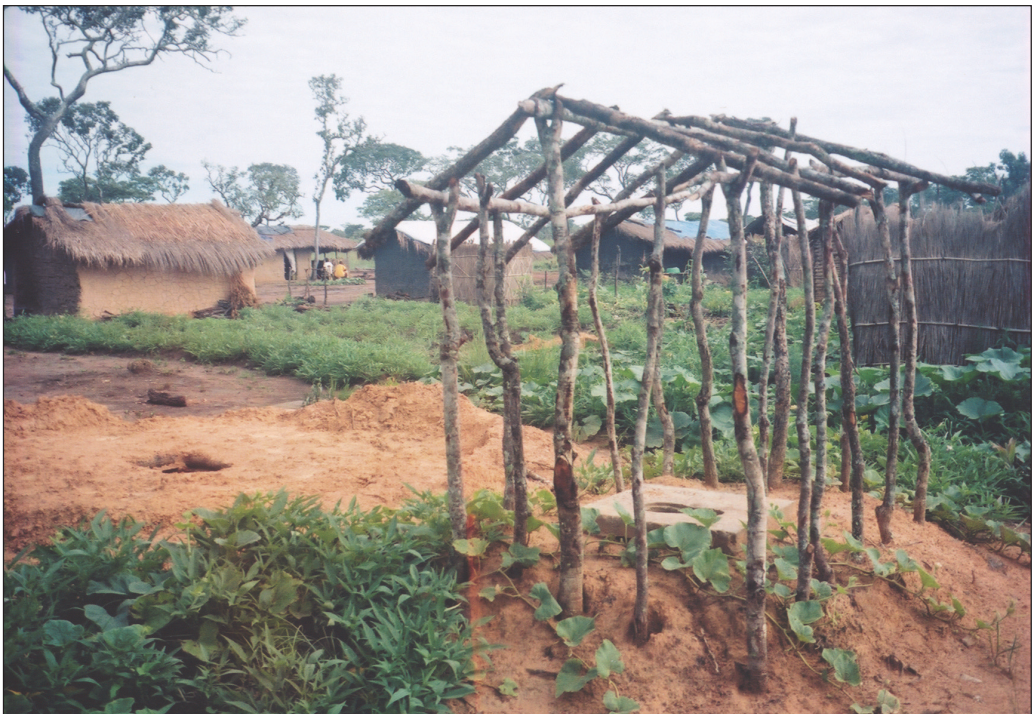
Family pit latrine under construction
