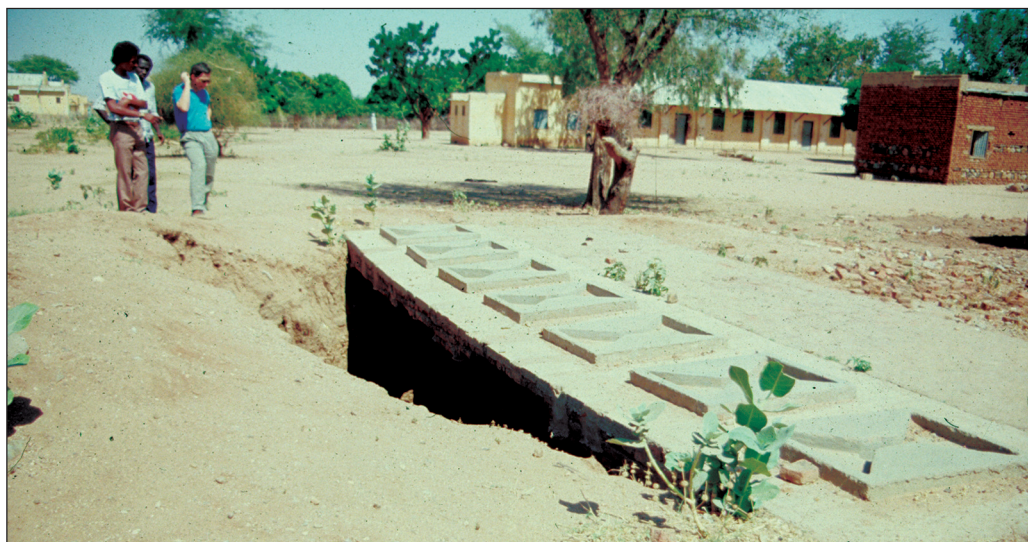
Failed unlined trench latrines, Sudan
