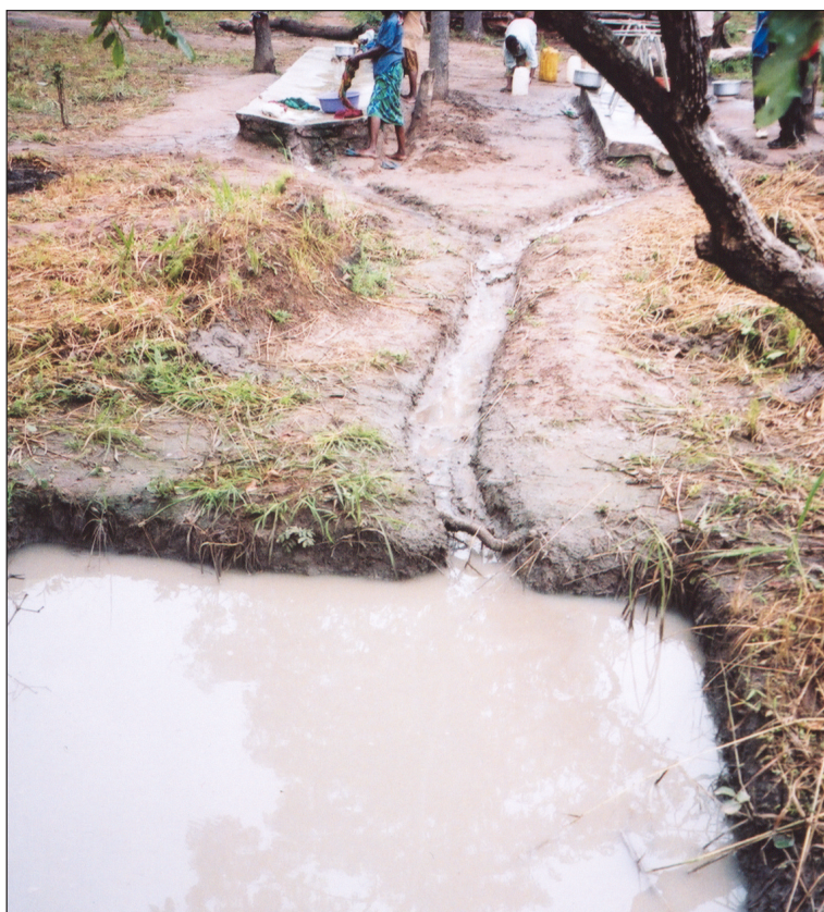
Poorly designed soakpit, Tanzania
