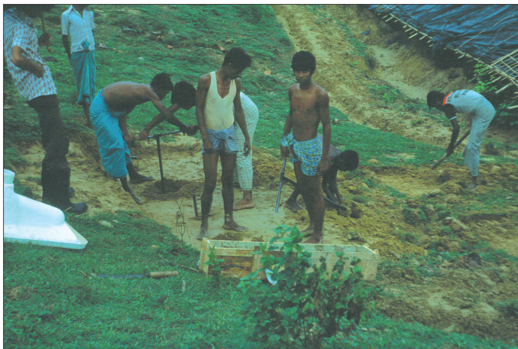
Drilling boreholes for latrines, Bangladesh
