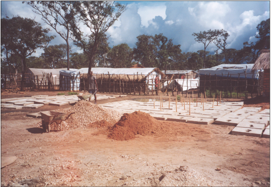
Preparation of concrete latrine slabs
