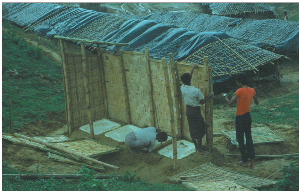
Borehole latrines nearing completion, Bangladesh
