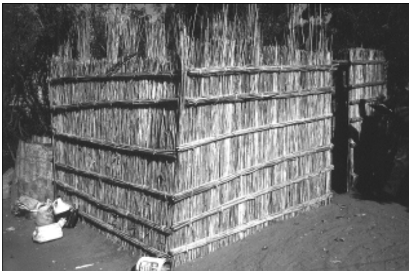
Photograph 1: Typical latrine superstructure (made from reeds) used in Mozambique, where it is customary for latrine shelters to be built without a roof
