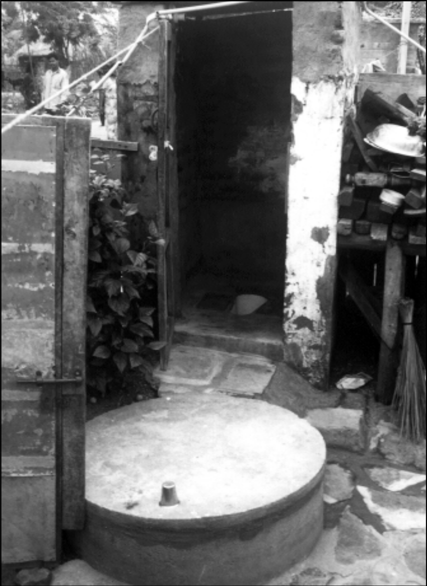
Photograph 4: Pour flush latrine in improved urban slum, Vijayawada, India. Operational sanitation facilities were found to be commonplace on the smallest of plot sizes (as small as 14m 2 )
