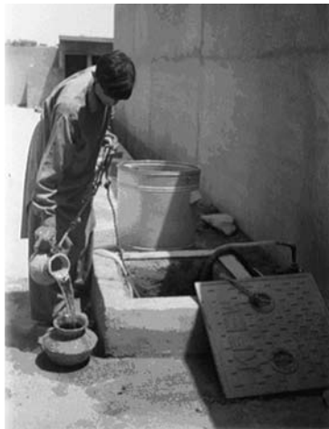
Photograph 5.1. A young man filling the pail of a household from an awami tank in Siddiq-e-Akbar Mosque, Gulshan-e-Zia, sector 11.5, Orangi Town. Nozzle of water motor is visible
