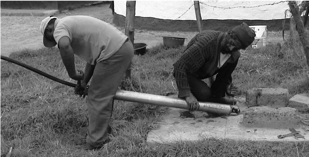
*Photograph 7.2. APM undertaking Vergnet pump repairs*
