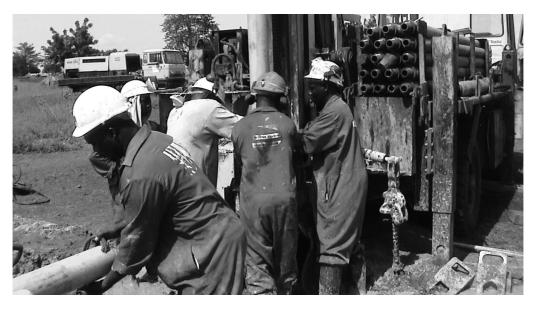
Photograph 6.3. Installing uPVC casing and screening in a newly drilled borehole
