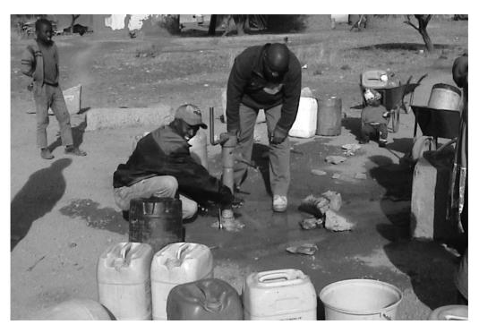
Photograph 7.3. Contractor undertaking maintenance on a Mono pump in South Africa
