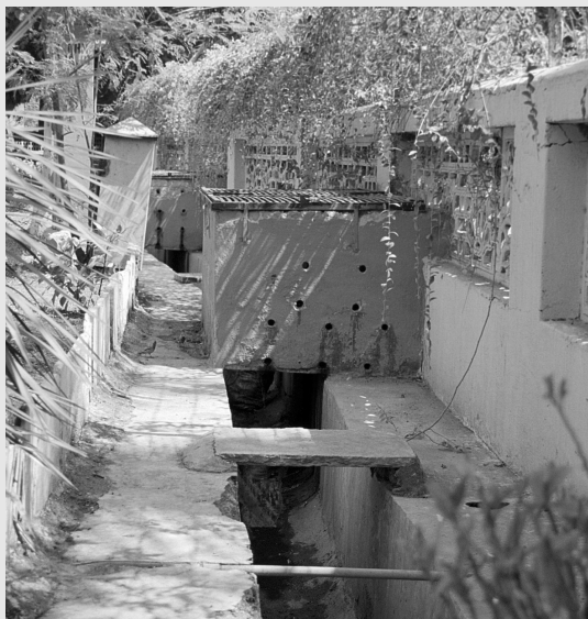
Photograph 3.3. Box system located at the Diamond Garden Residents Forum, treating the waste of 125 households. The compost produced is used for the greening of public places and as potting material. The bins are located above a drainage system at the former dumping area, which saves space. The neighbour appreciated the composting bins which replaced a smelly temporary dumping area.
