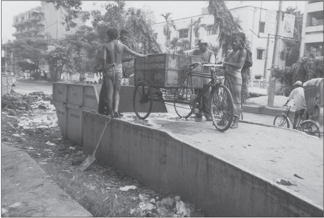
Ramp transfer system in Khulna, Bangladesh
