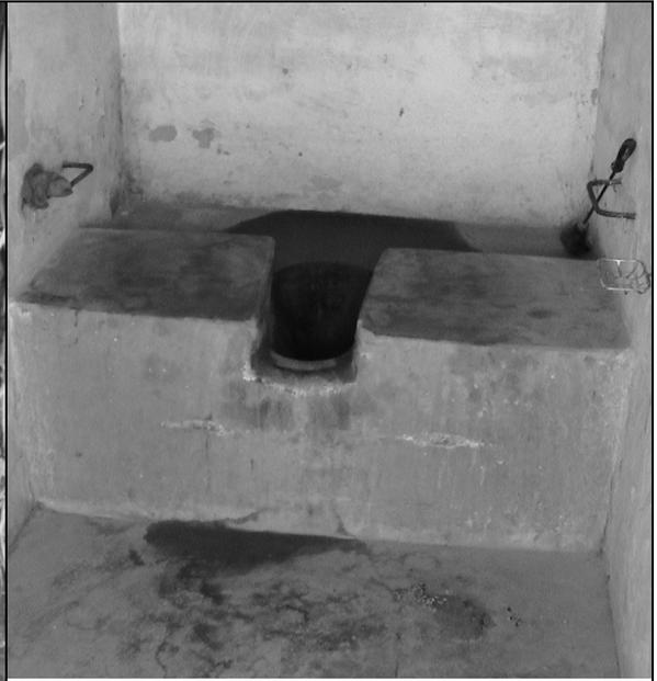
**Fig. 10: Raised concrete toilet platform**
