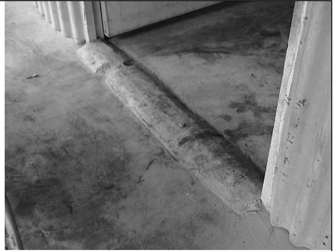
**Fig. 6: Rounded concrete threshold**
