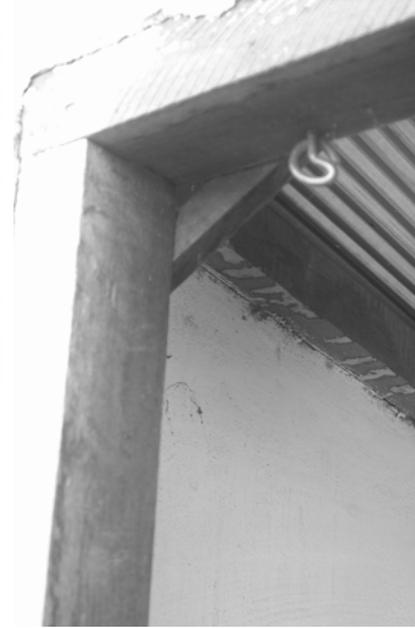
**Figure 15. Hook for running string through to shut toilet door (HI/CABDIC).**
