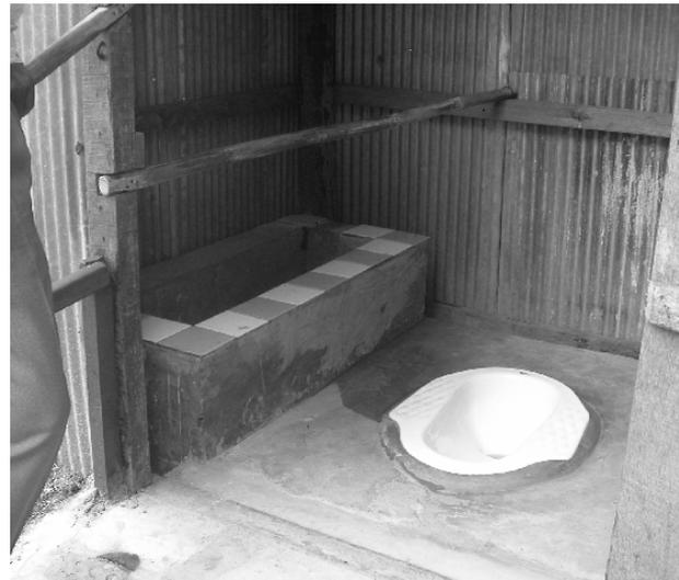
**Figure 17. Wooden handrail beside toilet extends from door to back wall (HI/CABDIC).**
