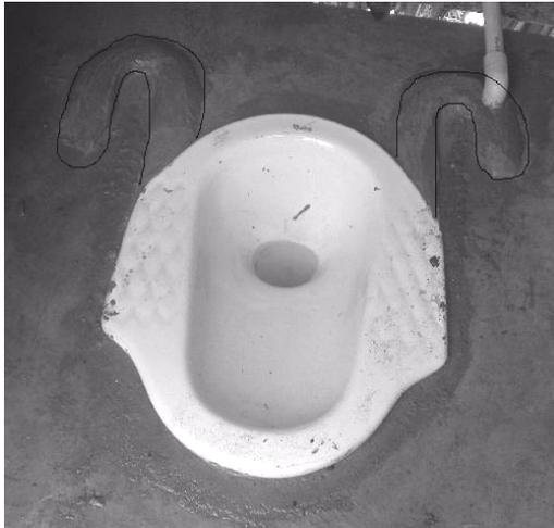
**Figure 20. Cement mouldings provide correct wheelchair positioning (CABDIC/HI).**
