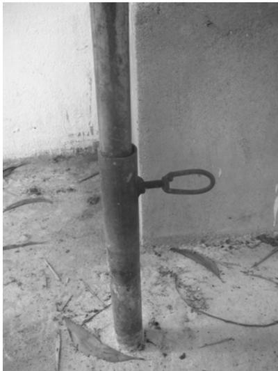
**Figure 16. Adjustable handrail made of iron pipe (HI/CABDIC).**
