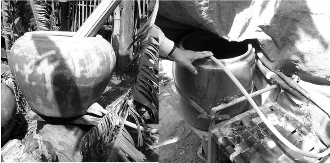
**Figure 9. Gravity fed system: hose from large rainwater storage jar leads to small jar in bathing area.**
