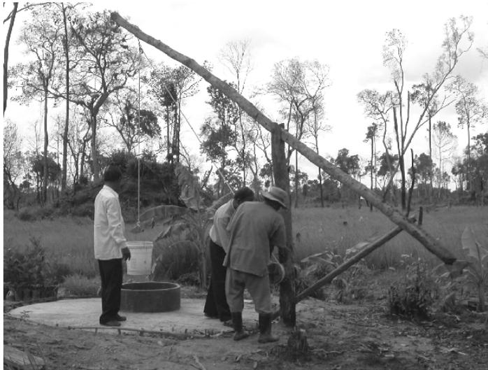
**Figure 4. Mr Ath Vuth demonstrates the fixed cantilever well that he designed and constructed himself.**
