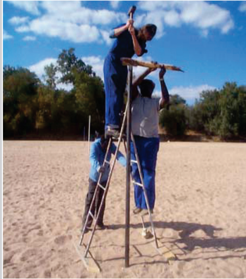
Photograph 5.6. Driving in a well-point to 3 metres
