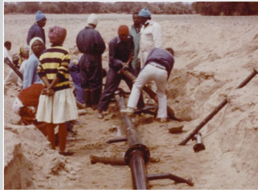
Photograph 5.4. Installation of a multiple well-point system
