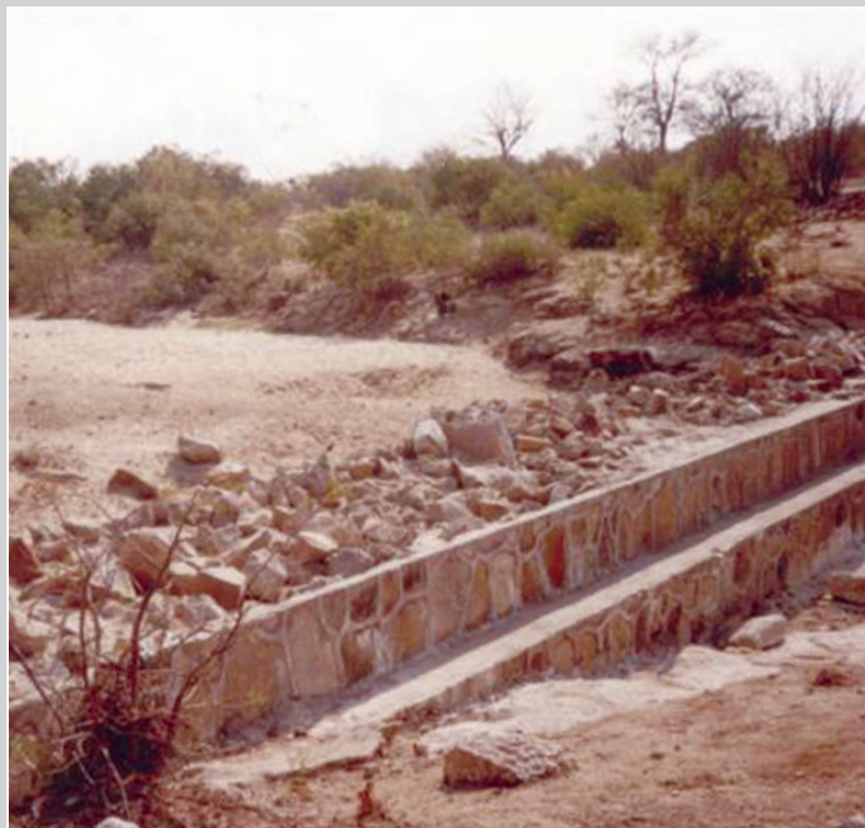
Photograph 4.10. Mkayi Wokhoza sand dam under construction
