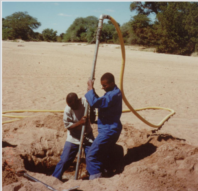
Photograph 5.8. Installing a self-jetting well-point
