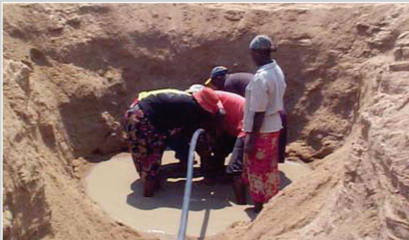
Photograph 5.5. Digging in a well-point
