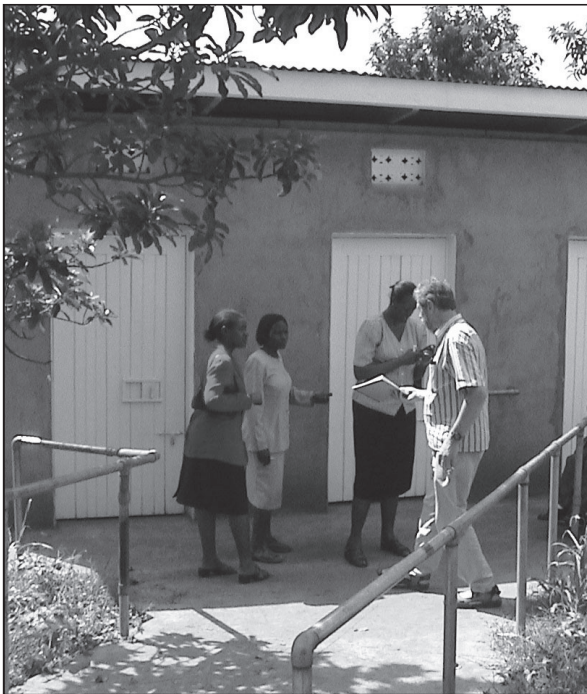
Figure 5.10. Wide concrete ramp with handrails both sides.
