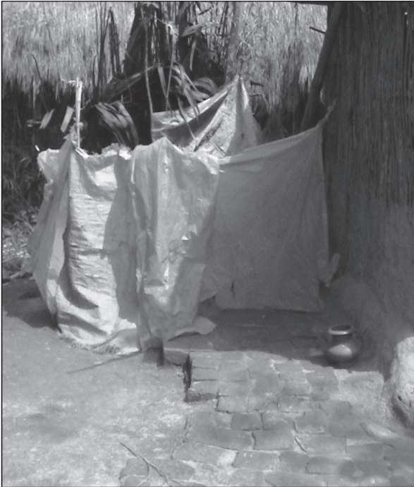
Figure 5.8. Brick path with earth and sand pointing leading to a bathing area.
