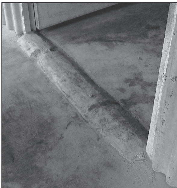
Figure 5.14. Low threshold for flood prevention, rounded for easy wheelchair access.
