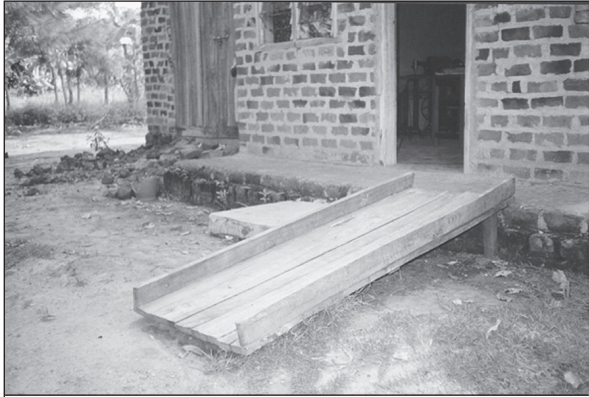
Figure 5.12. Movable wooden ramp.
