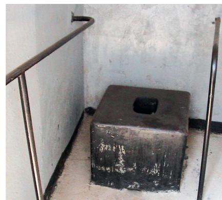
Figure 7. Raised toilet seat with rails fixed to wall and floor <sup>6</sup>
