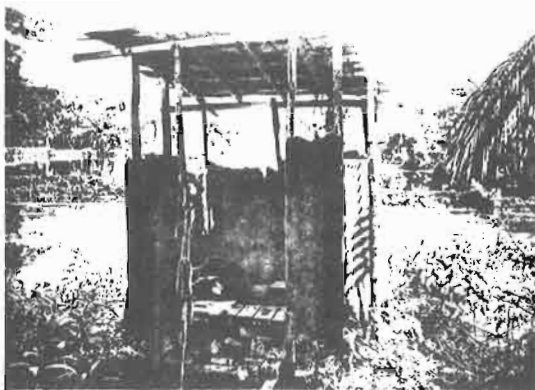
Latrine superstructure over a ditch.
