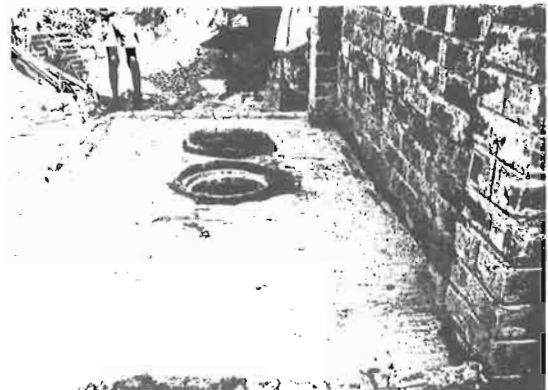
Sanitary latrine under construction.
