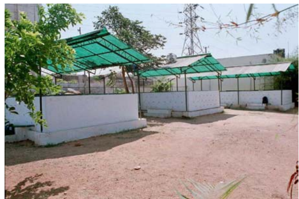
Figure 1. Composting bins at Kalyana Nagar, Banaglore
