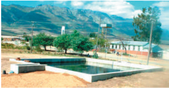
Figure 2. Slow sand filter in Tulbagh
