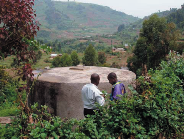
Photograph 1. A service reservoir in a 12 year old gravity flow scheme
