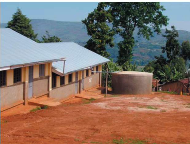
Photograph 2. Rainwater catchment at a primary school
