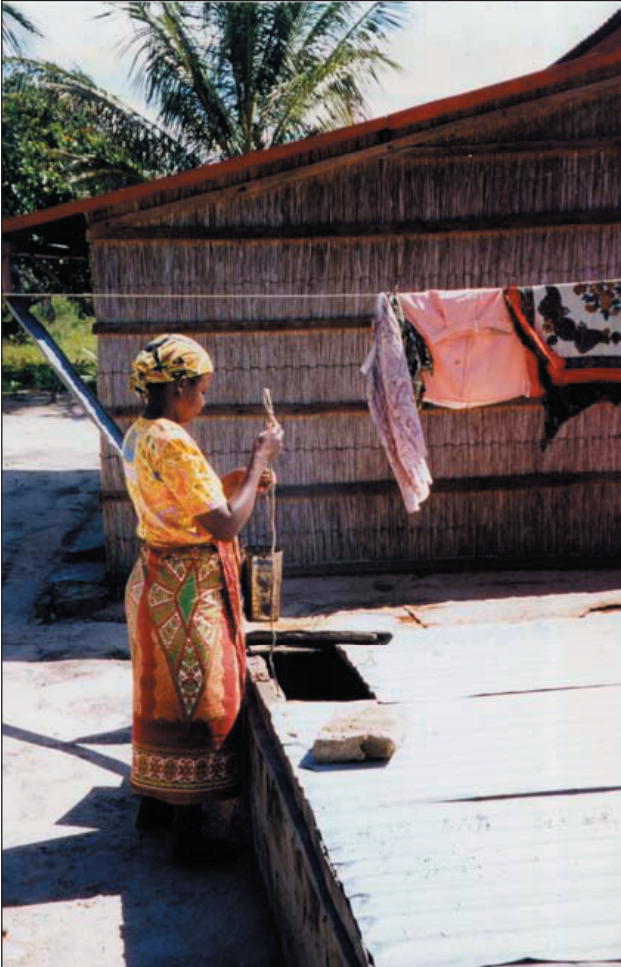
Photograph 1. Household RWH system, Inhambane, Moçambique
