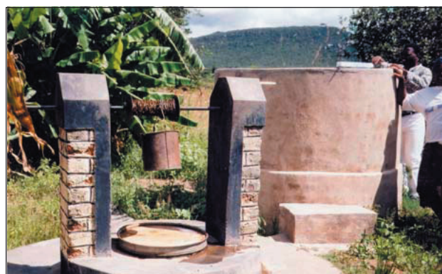
Photograph 2. Zimbabwe improved well, with cistern for irrigation
