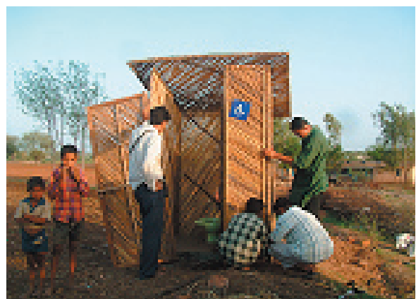
Photograph 2. A low cost DFT being constructed
