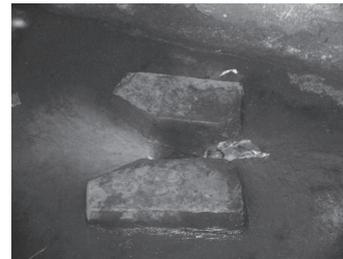
**Photograph 3. Inappropriate design (raised footplates)**
