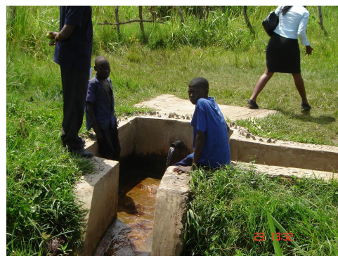
Photograph 2. A community spring in Amuria district. Community contributed land, sand, stones, labour, delivery pipe and fencing
