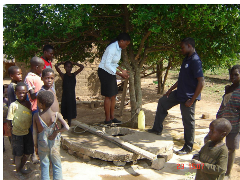
Photograph 1. A private well in Amuria district. Deepened, brick lined and covered on top in preparation for a hand pump
