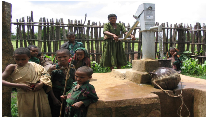
Photograph 1. WEDC – A woman fetching water from a dug-well fitted with Afridev hand pump
