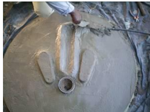
Photograph 4. A new well is made covered with cement and a rope pump. Total cost ca 600 US$
