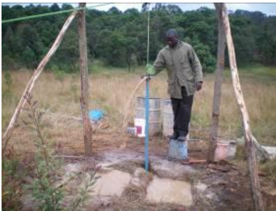
Photograph 1. Tanzania. Manual drilling of a 40 m deep borehole with the Baptist drilling technique
