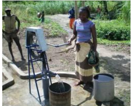
Photograph 4. A new well is made covered with cement and a rope pump. Total cost ca 600 US$
