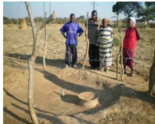
Photograph 2. Tube recharge system made by this family. Installed near a hand dug well
