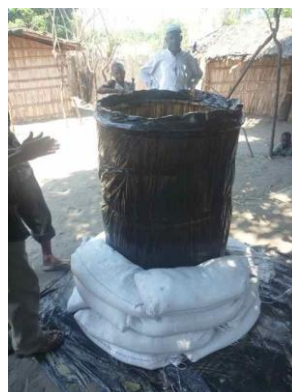
Photograph 3: Wooden frame (nkhokwe) is wrapped in plastic and reinforced with sand-bags
