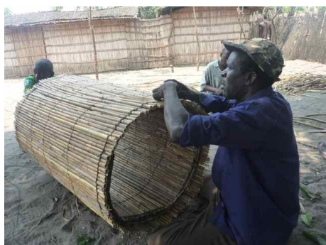
Photograph 2: Wooden frame (nkhokwe) is constructed using local reeds woven with rubber threads taken from tyres
