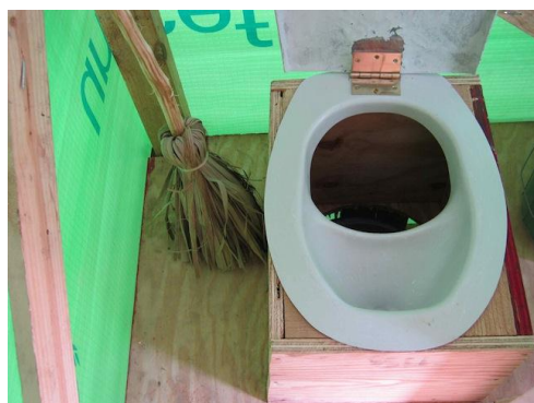
Photograph 3. Fibreglass UD seat made in Port au Prince
