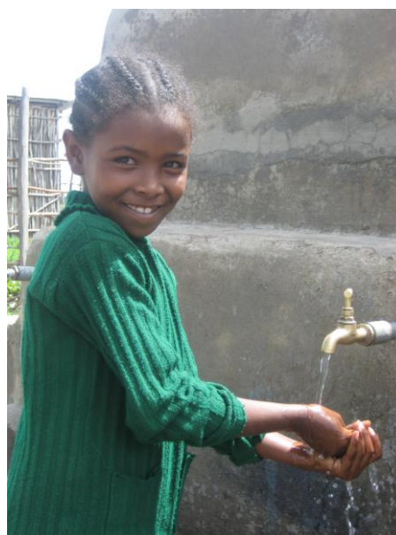
Photograph 3. A young student washes her hands at the newly installed multi-tap hand washing facility adjacent to the well with elevated hand pump
