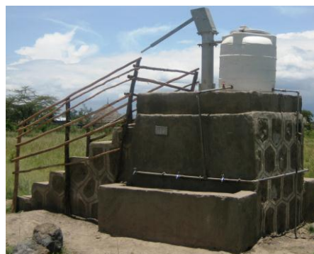
Photograph 1. Elevated hand pump with 250L storage tank and multi-tap hand washing facility at Weja Bati Primary School
