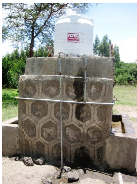
Photograph 2. Gravity fed pipe system, front view
