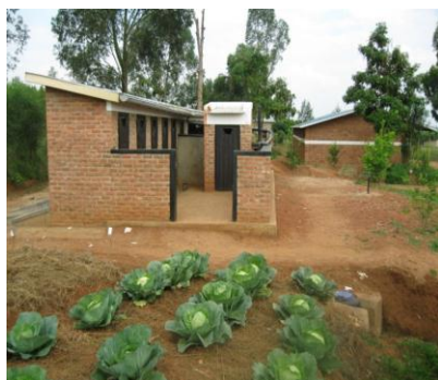
Photograph 1. WEDC - - Eco – San toilet
