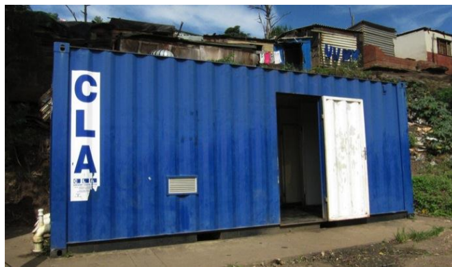
Photograph 1. Community ablution block in an informal settlement near Durban, South Africa
