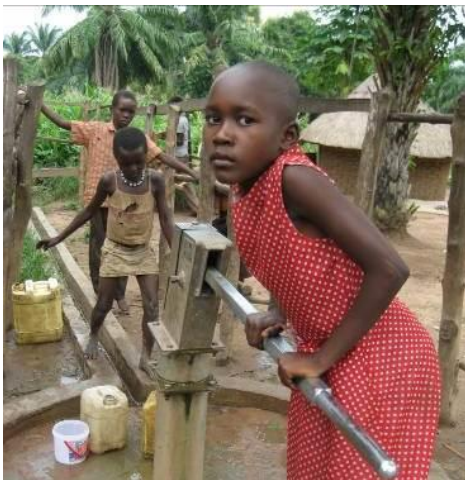
Photograph 1. Community borehole in Western Equatoria State
