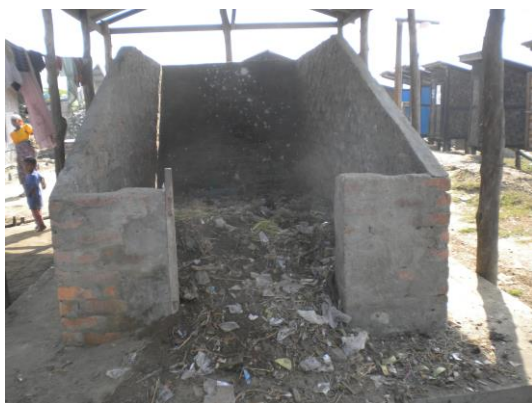
Photograph 1. Three-sided concrete collection point in OTG1
