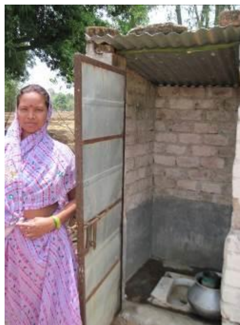
Photograph 8. Crampy Leach Pit Toilet
