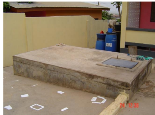
Photograph 2. Water storage facilities
