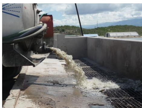
Photograph 1. Private pumper truck disposing of faecal sludge at Morne à Cabri WSP, November 2014
