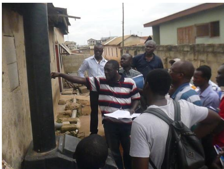
Photograph 1. Training of artisans in toilet construction
