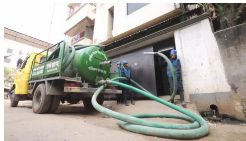
Photograph 5. MSEs emptying septic tank
