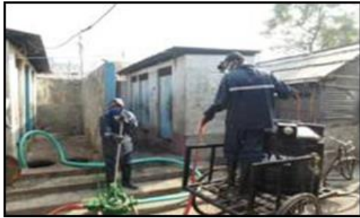
Photograph 2. SSEs emptying a septic tank
