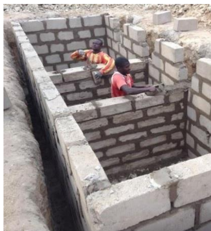
Photograph 2. CRS Ghana – pit of school latrine under construction
