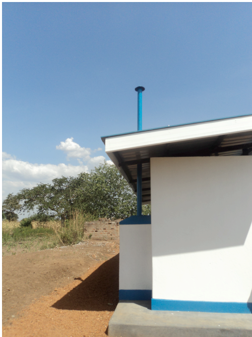
Photograph 1. A burning chamber attached to the washroom stance on a girl's latrine
