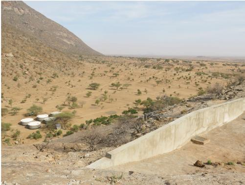
**Photograph 1. The completed rock catchment system Manyatta Lengima**
