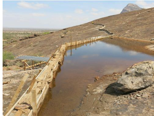
**Photograph 2. A almost completed weir of the rock catchment system in Ndikir**
