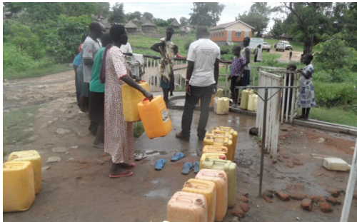
Photograph 1a. Borehole constructed in host community
