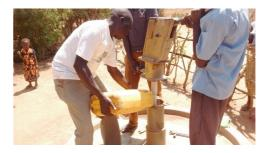
Photograph 2. HPM pouring 20 L of water mixed with chlorine into the borehole
