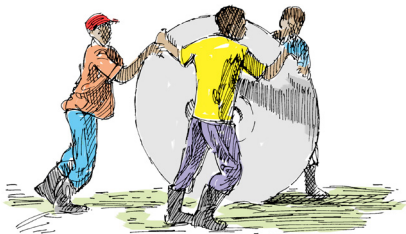
Figure 8. Circular slabs can be rolled into position, making them easier to move over short distances
