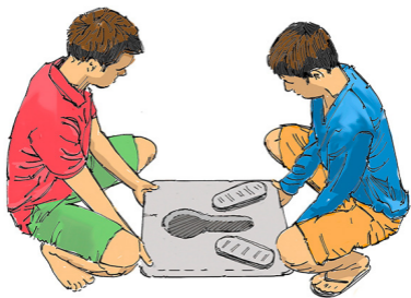
Figure 2. Lifting a sanplat into place
